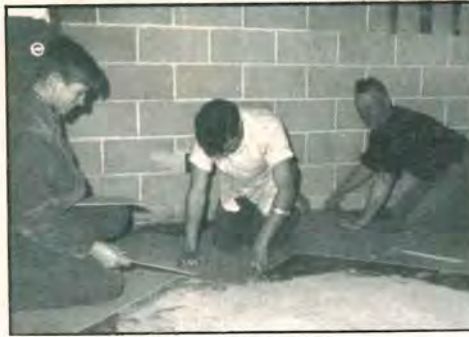
Youth help Larry Webb lay tiles on church's basement hall
